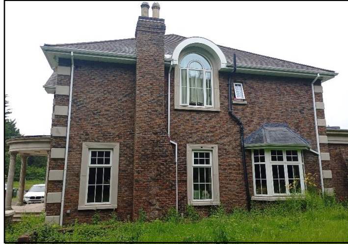
Plate 2: Existing building to be demolished (BL3)
