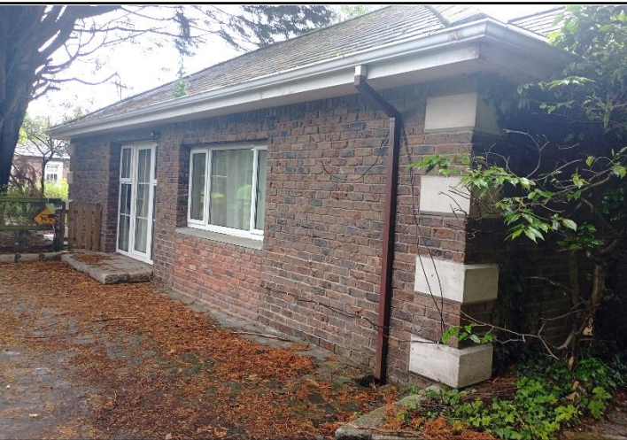
Plate 3: Existing building to be demolished (BL3)
